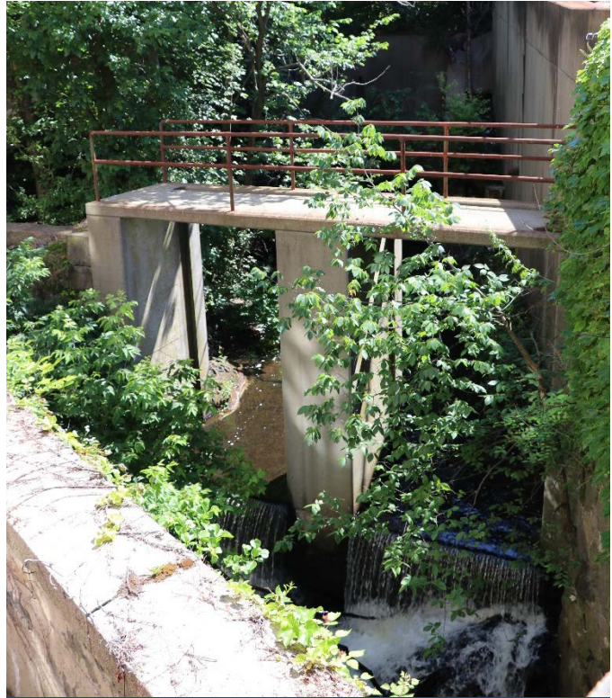
Figure 9. Short daylighted river segment above Mill No. 7
