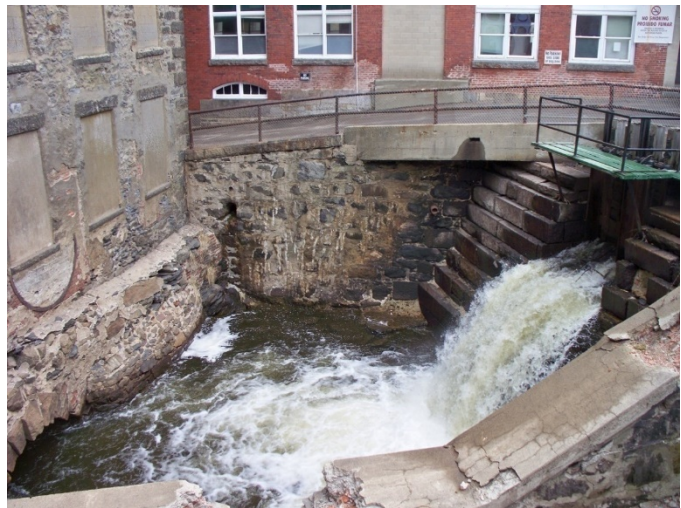
Figure 10. Spillway above Mill No. 6
