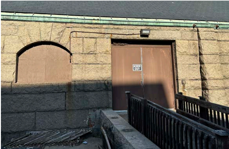
Figure 9 - Exterior Side (East Facing)
