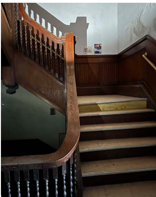
Figure 47 - First Floor (Stairwell)
