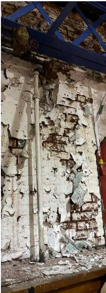
Figure 26 - Drill Hall (East)
