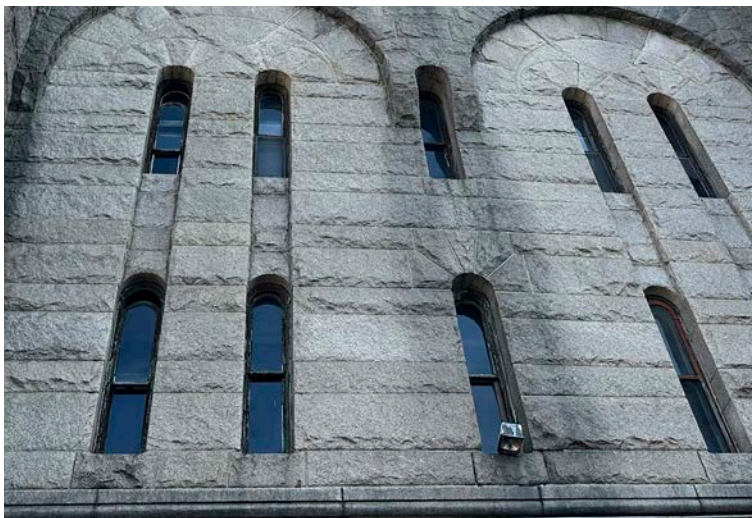
Figure 2 - Exterior Front (South Facing)
