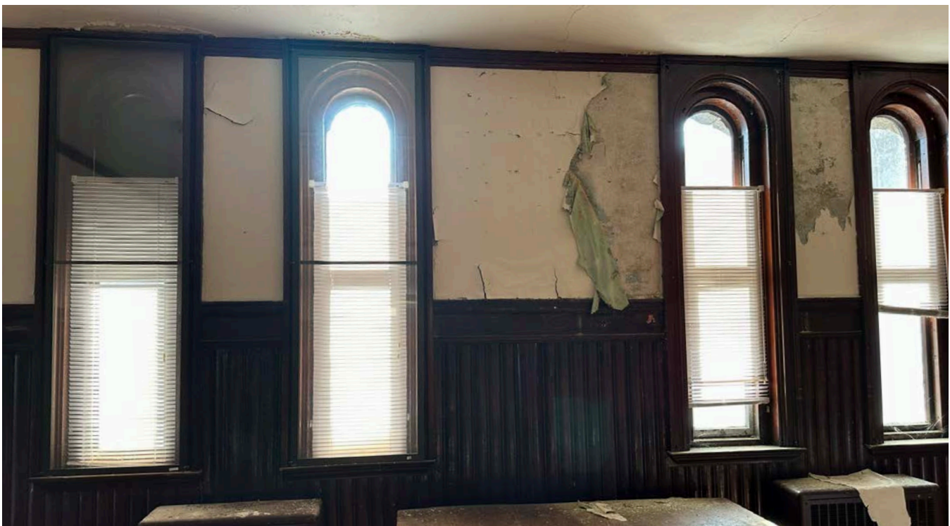
Figure 82 - Third Floor (East)
