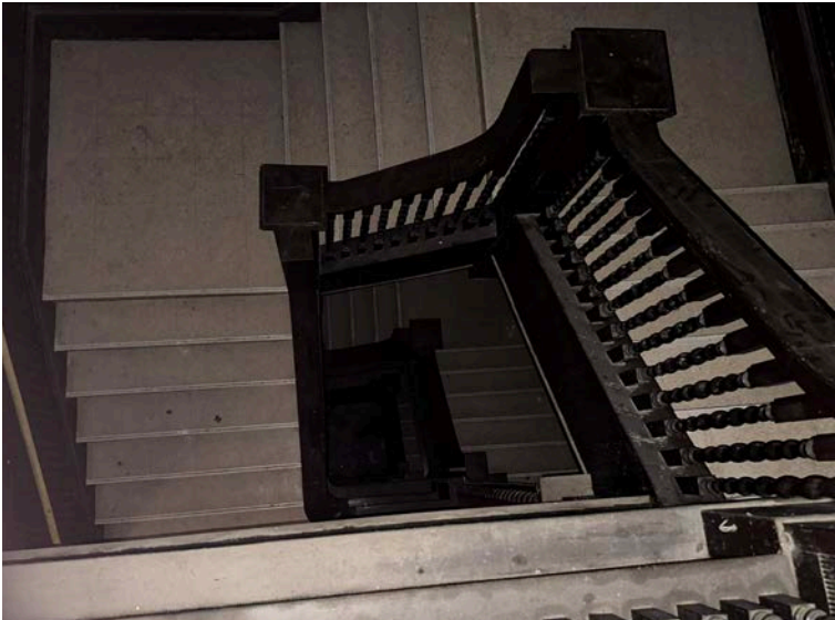
Figure 86 - Fourth Floor (Stairwell)
