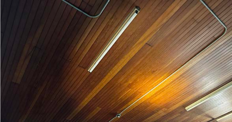
Figure 88 - Fourth Floor (Southwest Ceiling)
