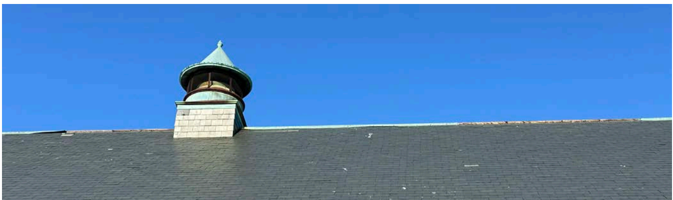
Figure 8 - Exterior Side (East Facing)
