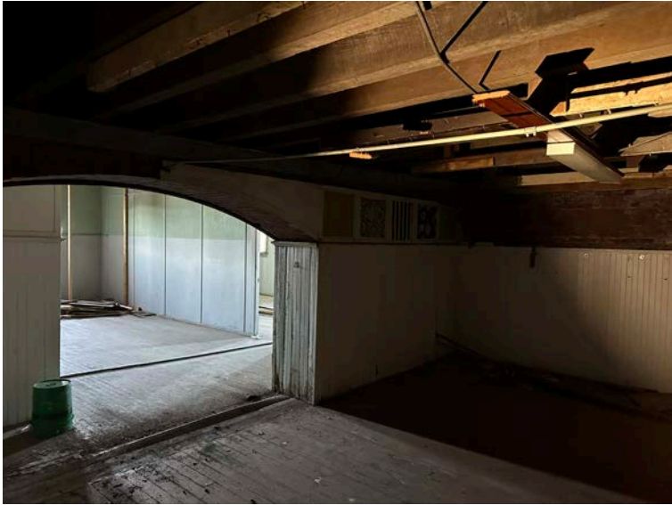
Figure 87 - Fourth Floor (Main Hallway)
