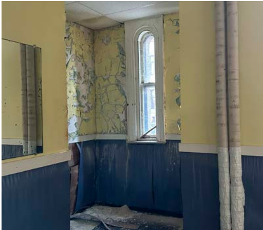
Figure 43 - First Floor (Southeast)
