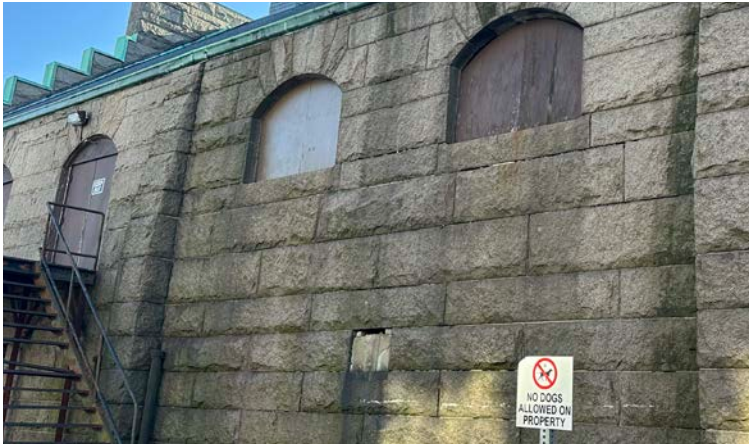
Figure 15 - Exterior Side (West Facing)
