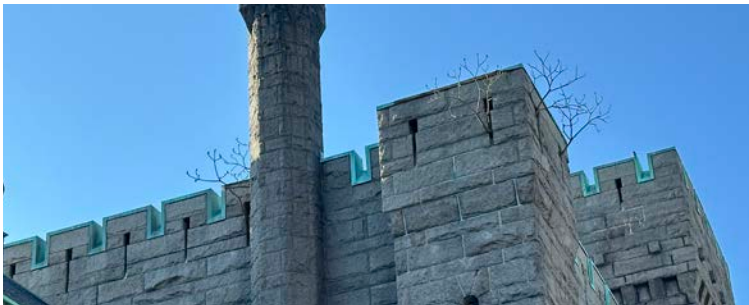
Figure 16 - Exterior Side (West Facing)
