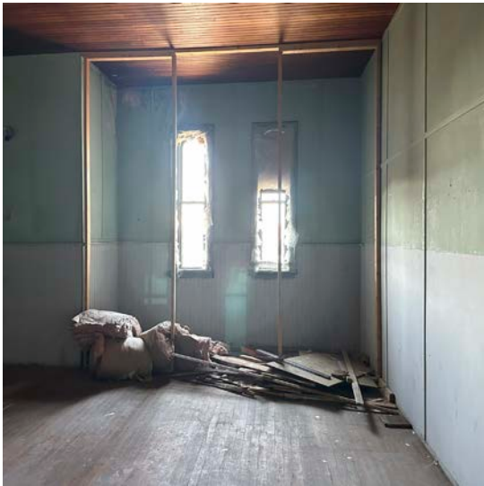
Figure 89 - Fourth Floor (Southwest)
