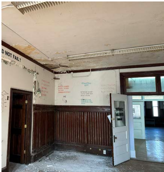
Figure 84 - Third Floor (East)
