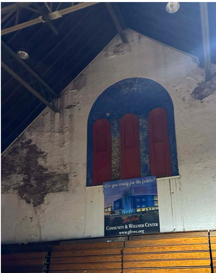
Figure 24 - Drill Hall (Rear)
