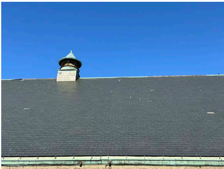
Figure 7 - Exterior Side (East Facing)
