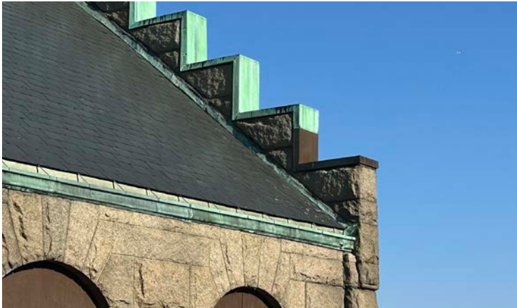
Figure 10 - Exterior Side (East Facing)
