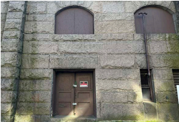
Figure 19 - Exterior Side (West Facing)
