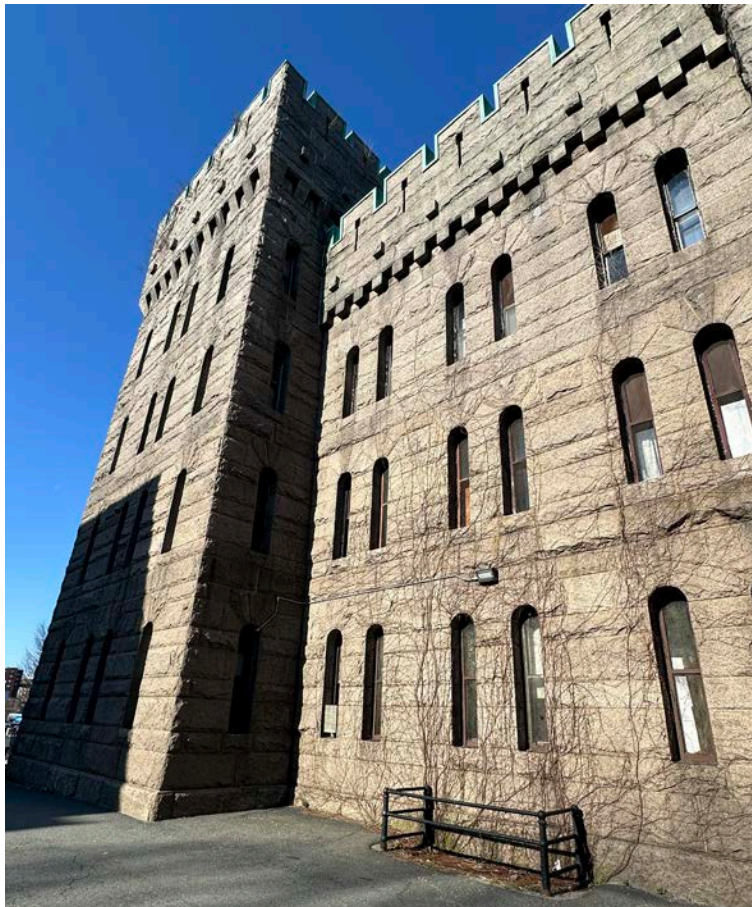
Figure 4 - Exterior Side (East Facing)
