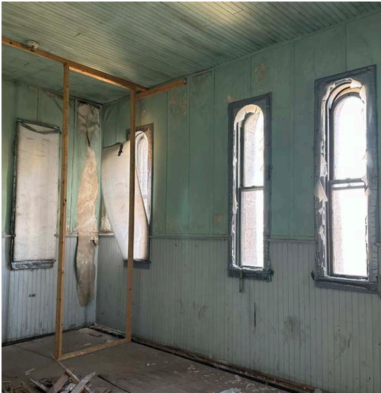
Figure 90 - Fourth Floor (Southwest)
