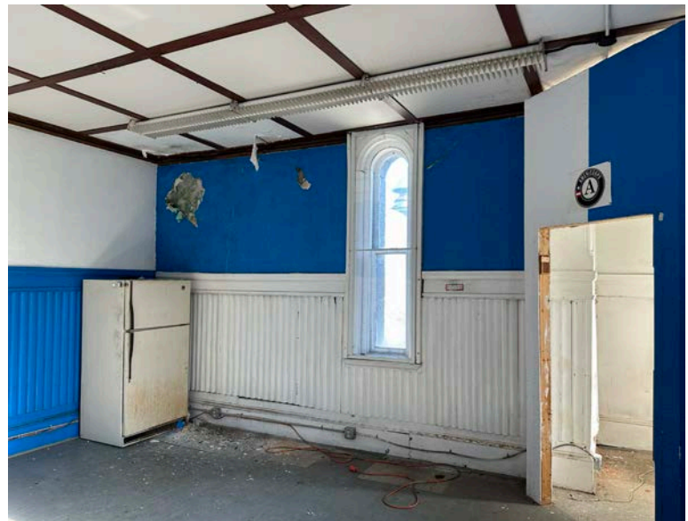
Figure 85 - Third Floor (East)
