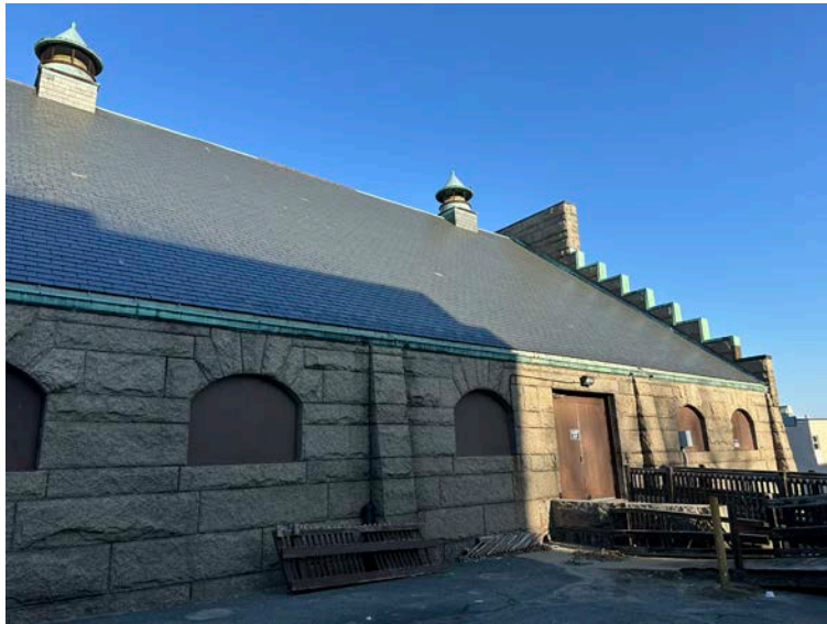
Figure 6 - Exterior Side (East Facing)
