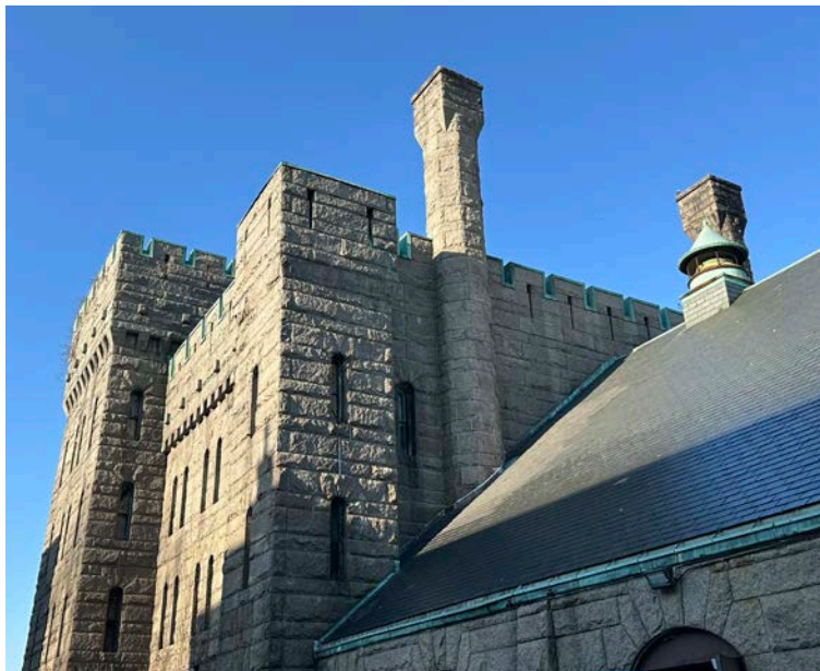
Figure 5 - Exterior Side (East Facing)
